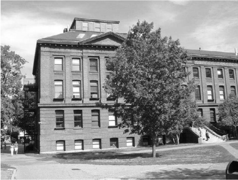
The west end of the Jefferson Physical Laboratory of Harvard University. The building was erected in 1884, including an inner tower, extending from the basement to the penthouse, which is isolated from the rest of the building. This tower housed the Pound–Rebka experiment.
